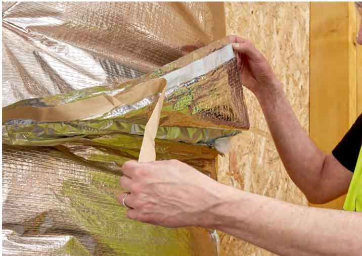
Butt-join **Eolis HC** with the next layer of the product. Peel back the paper from the built-in self-adhesive tape and bring the entire overlap in contact with the lower layer sealing securely. Vertical joints are to be sealed with **ACTIS** tape which is recommended for the product.
