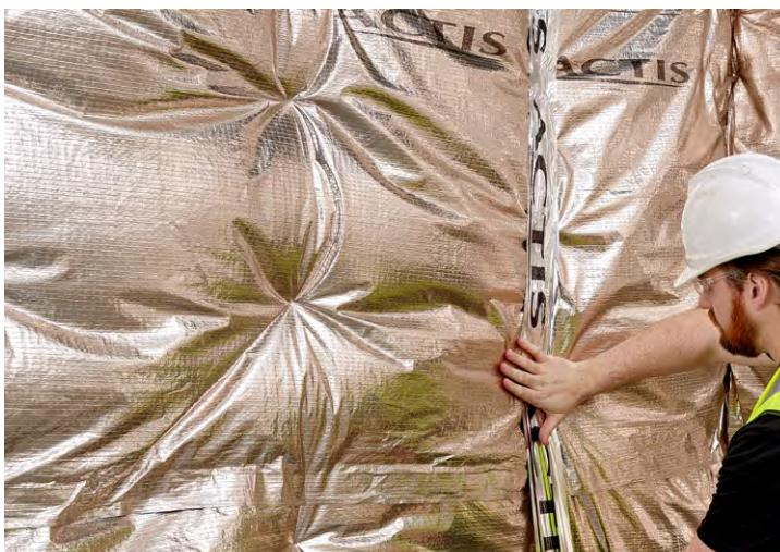
All perimeter edges, including around windows and doors should be stapled every 50mm and sealed with tape and secured by battens.
