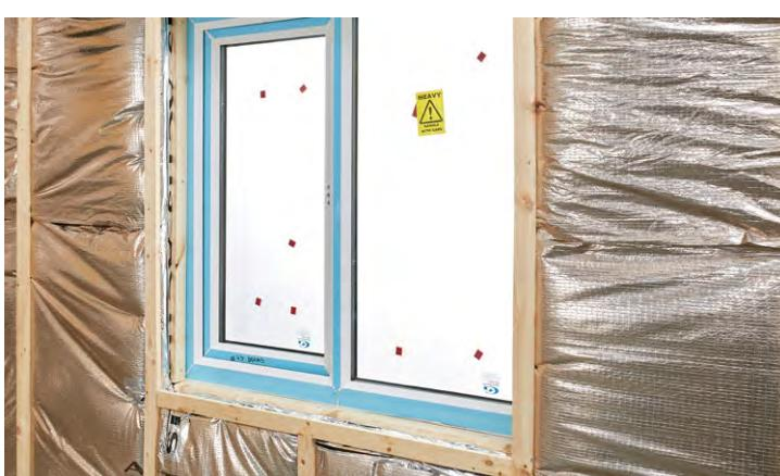
Around windows and doors, seal **Eolis HC** with **ACTIS** tape and secure with battens.
