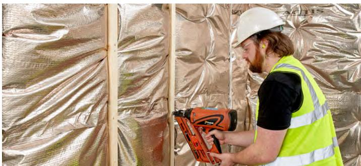
Prepare for plasterboard by fixing horizontal or vertical battens (size in accordance with specification e.g. 25mm, 38mm, 50mm battens) nailing or screwing through **Eolis HC** to timber structure. Where joints between plasterboard sheets are unsupported, timber noggin should be installed.
