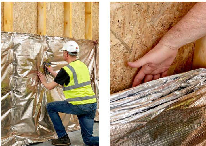
Install **Eolis HC** across the face of timbers fixing in a continuous layer. Maintain insulation thickness by making sure that the product is not pulled too taut and that the insulation fills the space required to accommodate product thickness. Maintain an air gap where required in accordance with your specification. Staple to timbers every 250mm, using min. 14mm galvanised staples.
