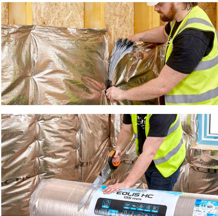
**Eolis HC** can easily be cut using an **ACTIS** cutter or a sharp knife. Align a timber batten where the product is fixed onto timbers and cut along pressing the timber batten firmly onto the product. Alternatively an electrical circular shear tool can be used.
